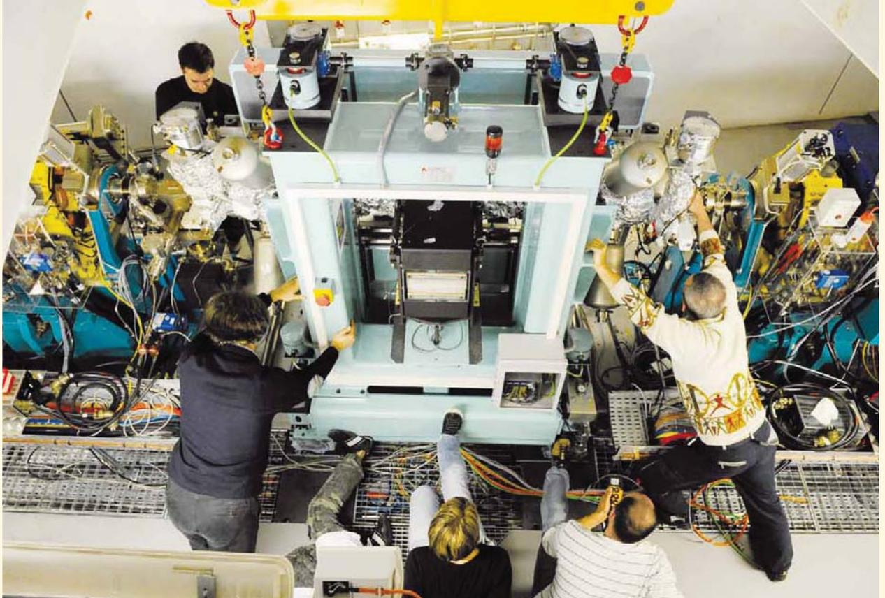
Installation of an undulator in the storage ring tunnel.
