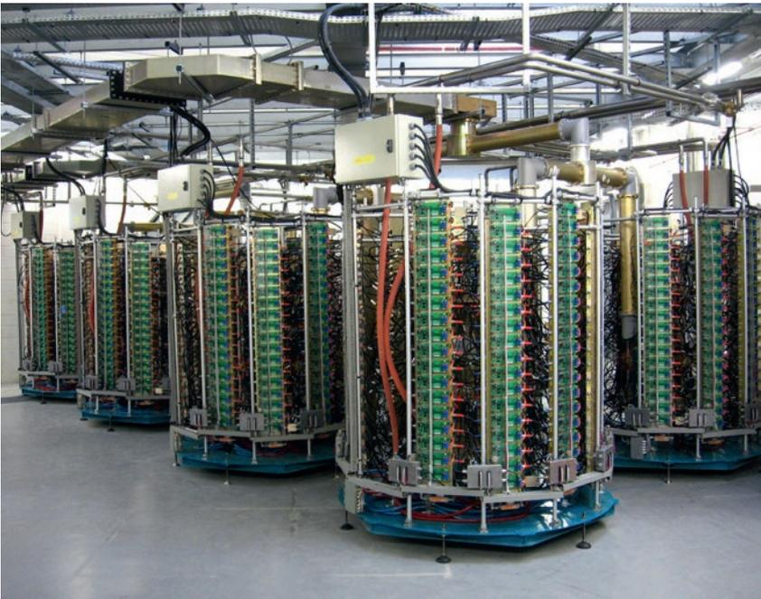
Figure 81: SOLEIL solid state amplifiers for the cavities 1 and 2
