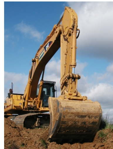
First dirt excavation on April 22, 2003
